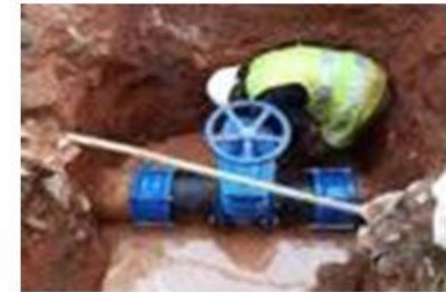
Valve installation on the trunk main
