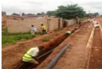
Pipe Laying within the DMA
