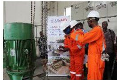
Overhauling of High lift Pumps
