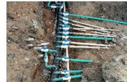
Reconnection of 105 Service Lines at Top Medical Point C
