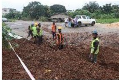
Laying of distribution pipes
