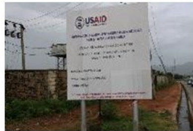
Construction activity signpost
