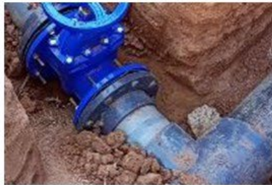
Laying of Control Valve on the line
