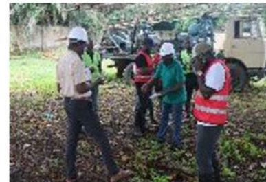
Identified locations for the borehole
