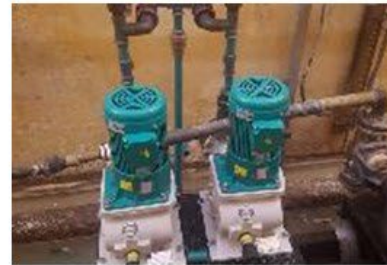
Dosing pump installation at the Chanchaga Water Works
