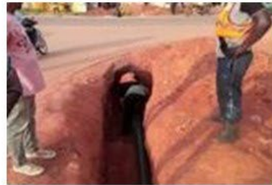
Thrust boring through a major road
