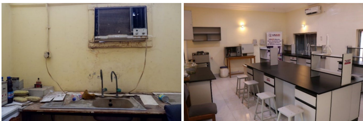
Left: Niger laboratory, 2019. Right: Renovated laboratory, 2021. Photos: USAID E-WASH.
