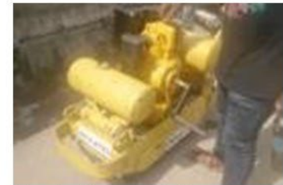
Hand roller on site for resurfacing of asphaltic road
