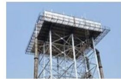
Rehabilitated 1,600 KVA Service Reservoir
