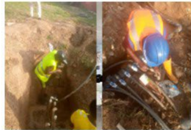
Service reconnection on distribution mains
