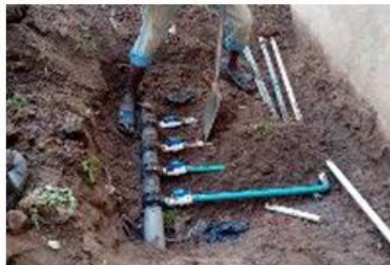
Reconnection of Service Lines at Barikin Saleh
