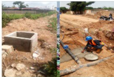
Construction of Valve chamber
