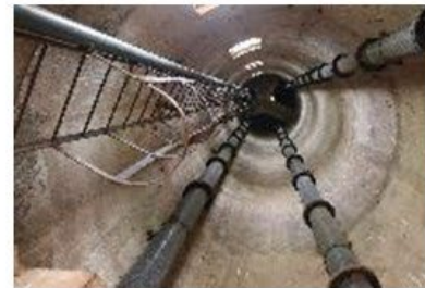
Elevated Concrete Tank
