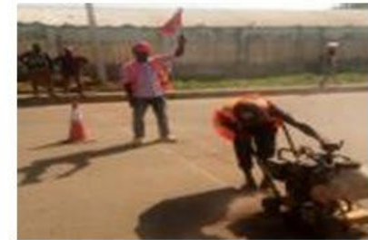
Road cutting for Pipelaying
