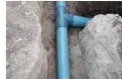
Installation of Tee on the pipeline
