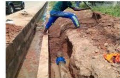
Repair of Leakages on DMA Network
