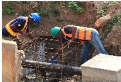
Disconnection/Reconnection of service pipes
