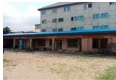
Rehabilitation of Staff-quarters
