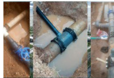
Laying of new distribution mains
