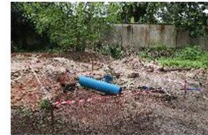
Cordoned area for piping works
