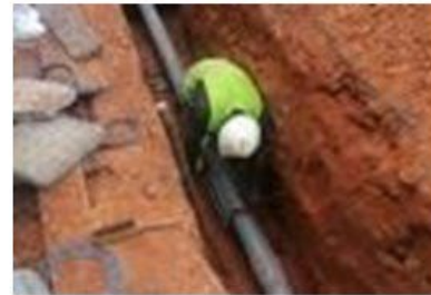
Connection point to the existing trunk main
