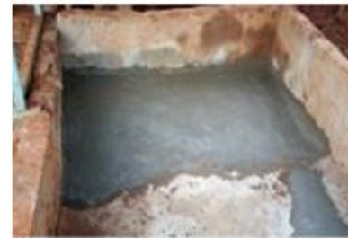
Reinstating pavement along Distribution Network
