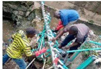
Reconnection of Service Lines at Kpakungu Bridge
