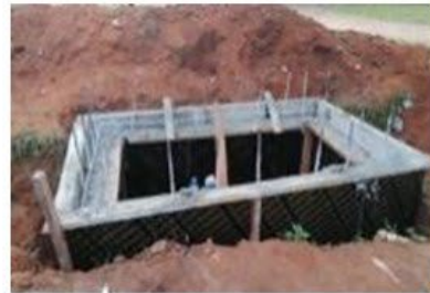
Valve chamber under construction
