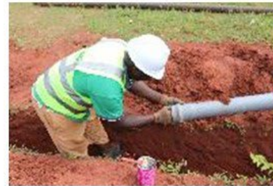
Laying of Distribution Pipeline
