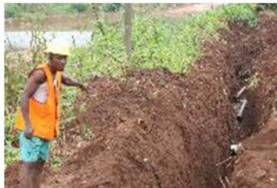
Distribution Pipeline Route Excavation
