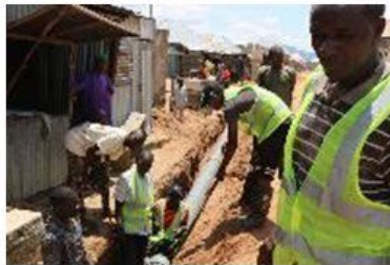
Pipe laying activity
