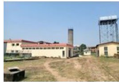
Overview of Renovated Office building
