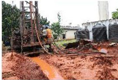
Drilling of new borehole
